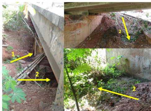
Figure 5. Flow at the Bottom of the Bridge
