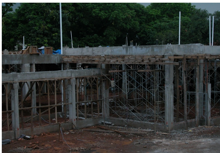
Fig. 10. Formwork
